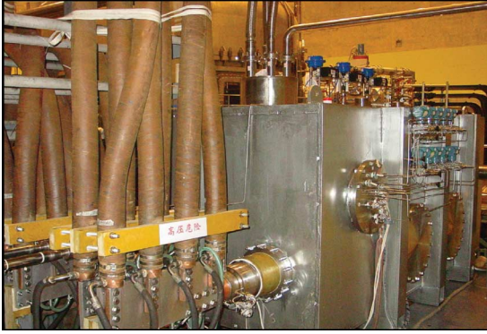
Fig. 14. HTS bus-bar for ITER.
